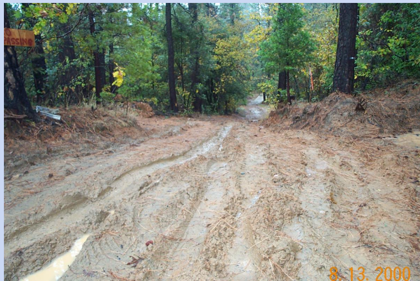
Ruts created by wet weather use of an unsurfaced, poorly drained road. Photo by Angela Wilson, Central Valley Regional Water Quality Control Board.
