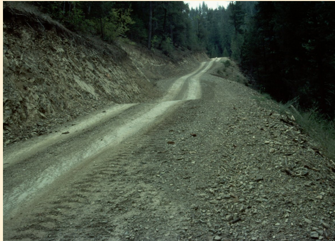
Rolling dips installed to drain an out-sloped road. Photo by Bill Weaver, Pacific Watershed Associates.
