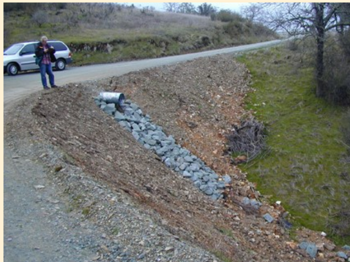
Rock armoring at ditch relief culvert outfall to reduce the potential for downstream erosion. Photo by Jared Gerstein.
