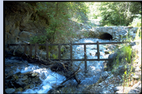
Trash rack installed upstream to protect the culvert from plugging. Photo by Keller and Sherar 2003.
