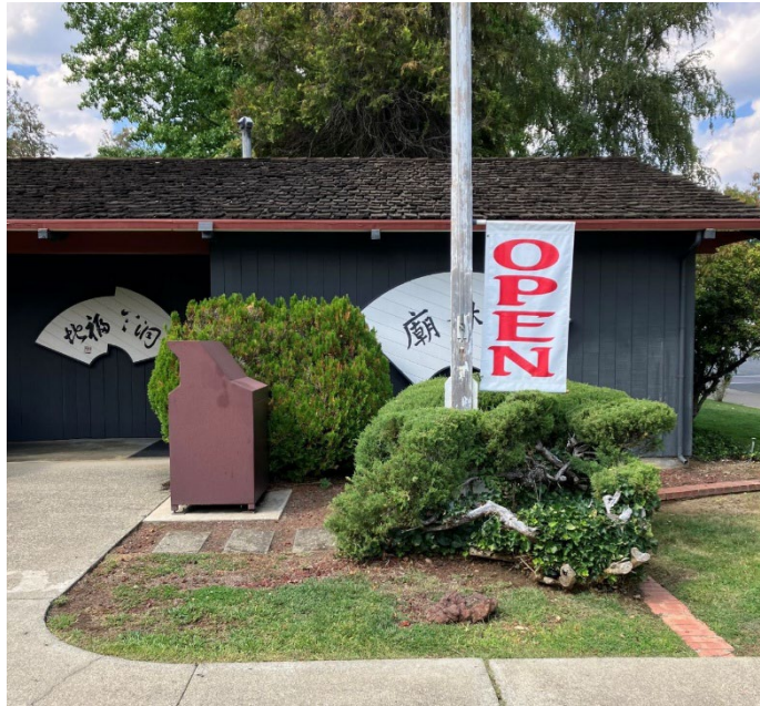
Figure 2. Existing condition, Area 1, unmodified photograph, September 2025.
