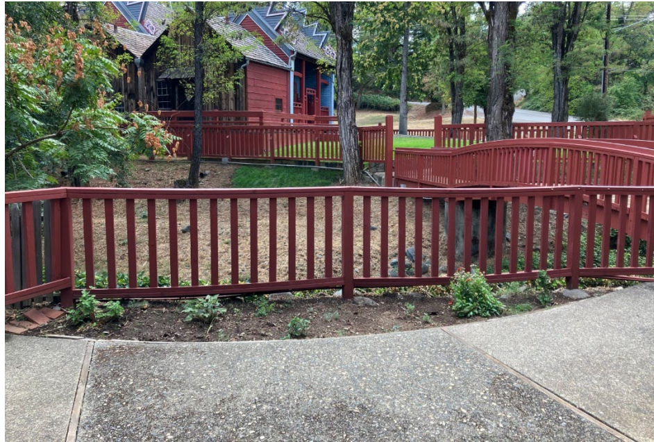
Figure 8. Existing condition, Area 3, unmodified photograph, September 2025.
