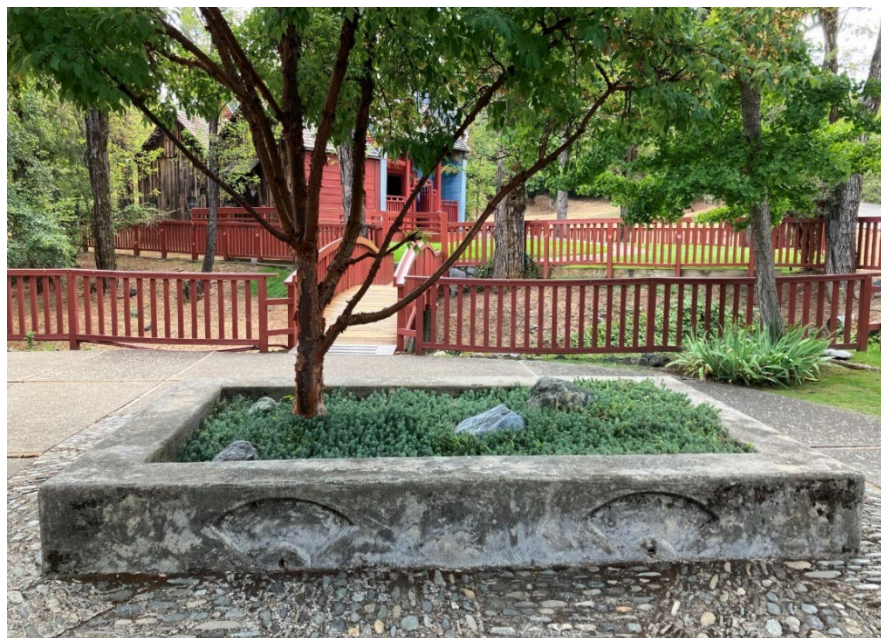
Figure 11. Existing condition, Area 4, unmodified photograph, September 2025.
