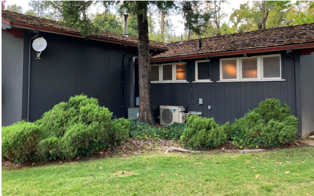
Figure 29. Existing condition, Area 9, unmodified photograph, September 2025.
