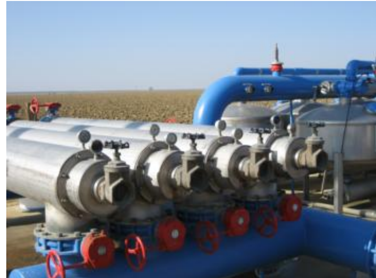
Screen filters used in conjunction with sand media filters. Photo L. Schwankl
