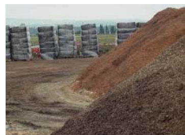
Soil piles lacking any protection from storm events.
