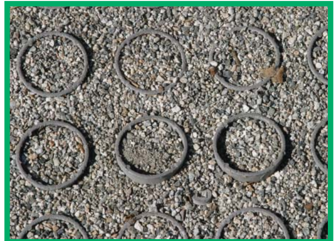
Example of plastic grids used to hold gravel applied to driveway entrance.
