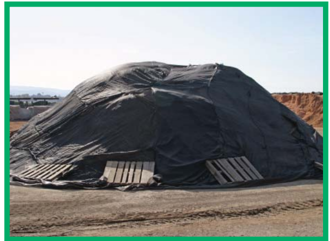
Example of soil pile covered with tarp to protect from wind and rain.
