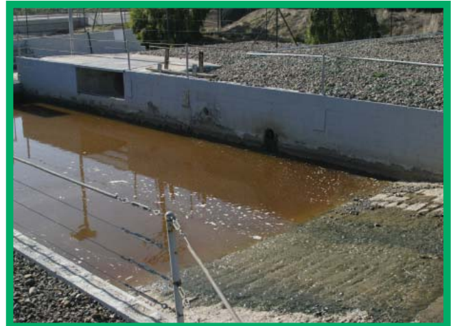
Example of a concrete water collection basin built wide enough to accommodate equipment to remove sediment.
