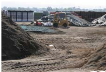
Soil piles lacking any protection from storm events.
