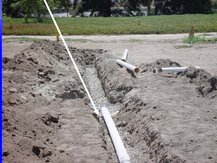
Perforated pipe covered with filter sock.
